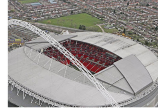
Wembley Stadium UK
